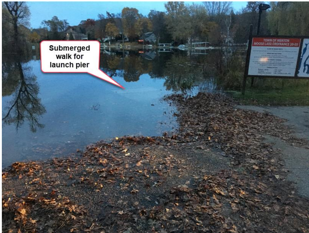
Flooded boat-launch southeast bay – October 31, 2018 Note concrete walkway under water leading to (removed) floating launch pier.
