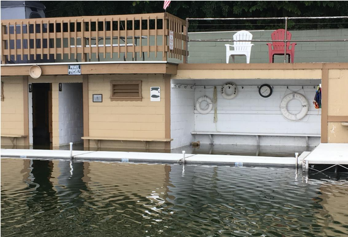
Flooding Carl Schurz Park swim platforms and changing rooms west shoreline - September 10, 2018
