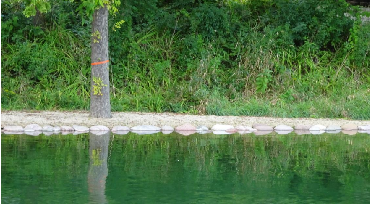
High water southeast bay, east side peninsula – August 30, 2018 Note erosion control stone rip-rap no longer effective height as to wave action.
