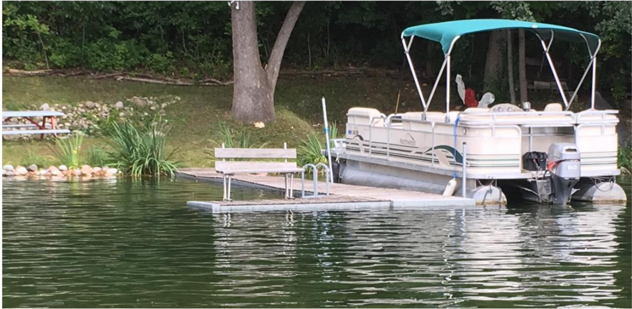
High water northeast shoreline – August 30, 2018 Note erosion control stone rip-rap no longer effective height as to wave action.
