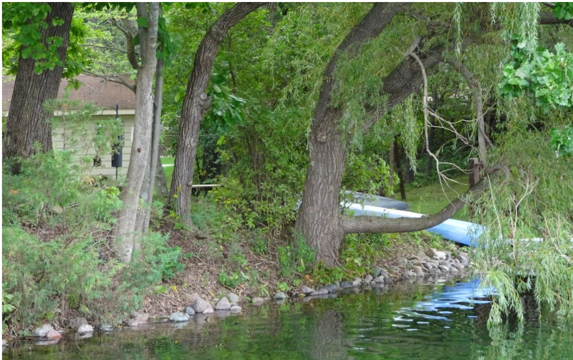
High water east shoreline – August 30, 2018 Note erosion control stone rip-rap no longer effective height as to wave action.
