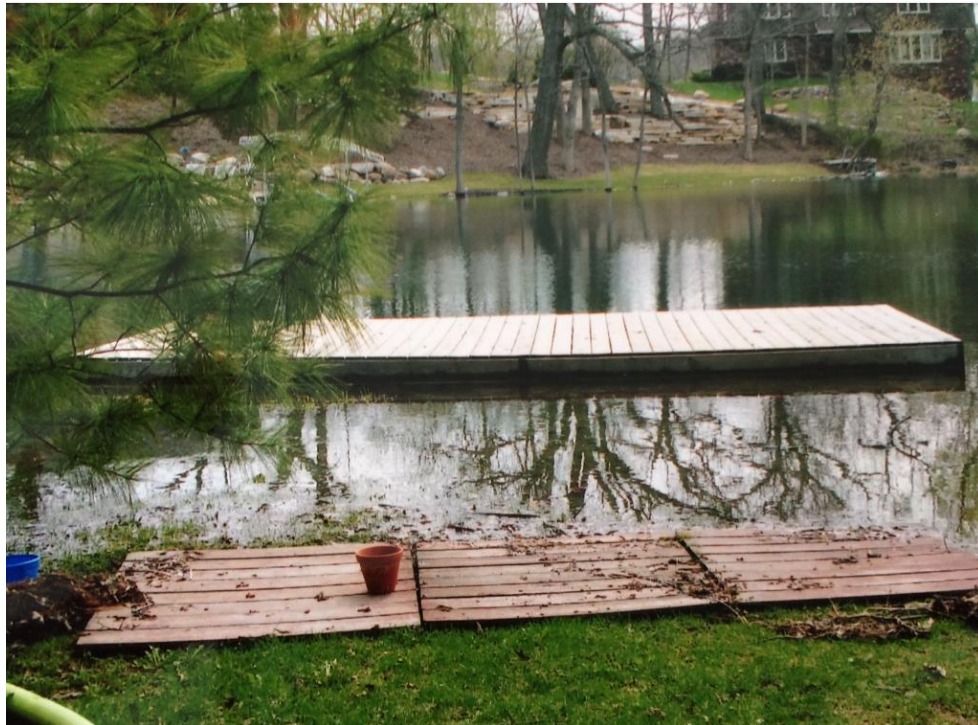
Tolbolski 2008 photo – pier and yard flooding southwest shoreline
