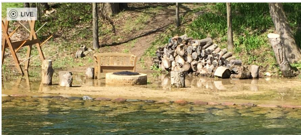
May 10, 2019 photo - Flooding east shore of peninsula. Shore rip-rap under water.
